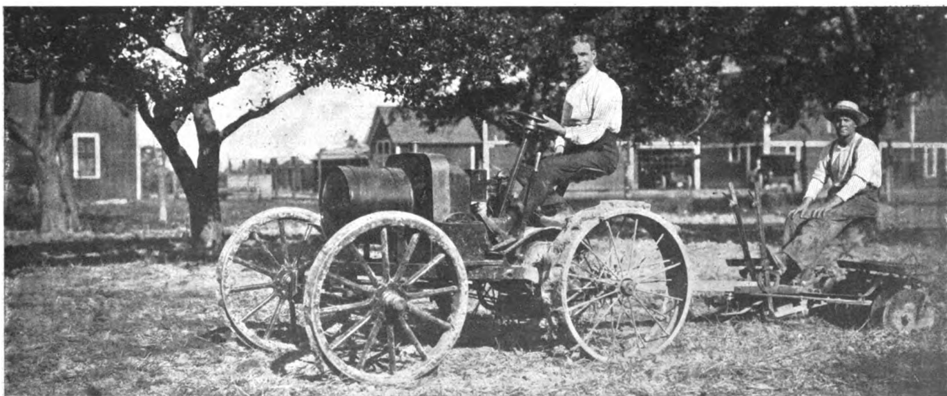
How Henry Ford Utilizes an Automobile Plow of His Own Design on His Farm Near Detroit.
